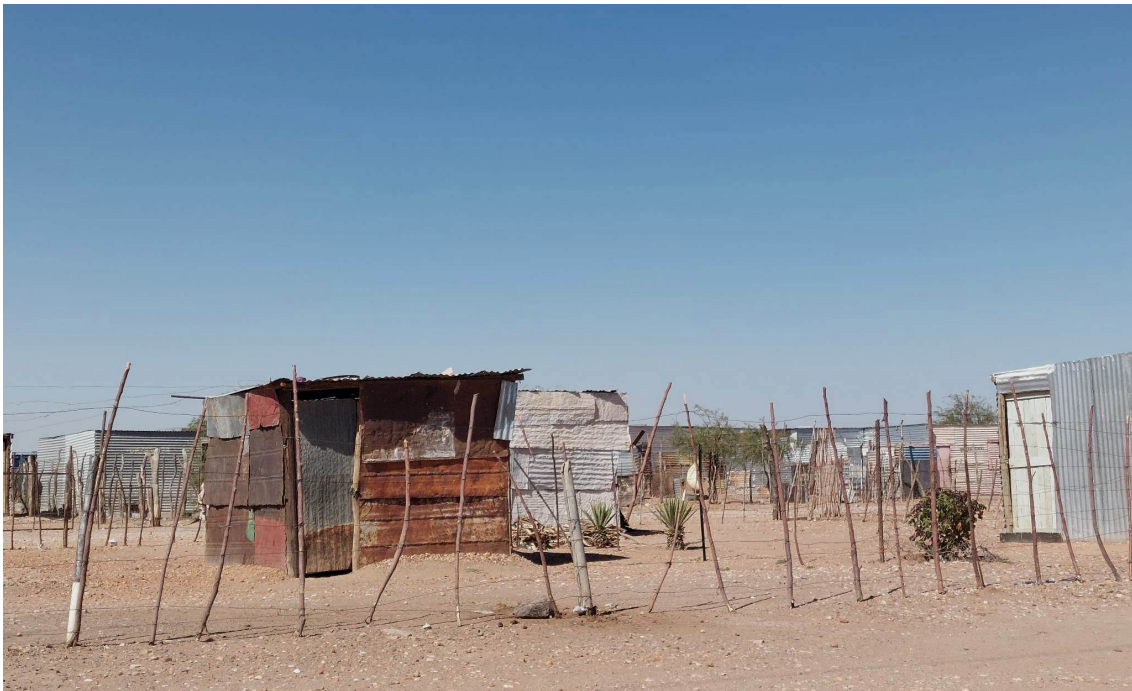
Photo 4: Informal settlement in Rehoboth. Illustrating the shacks that constitutes these areas.
